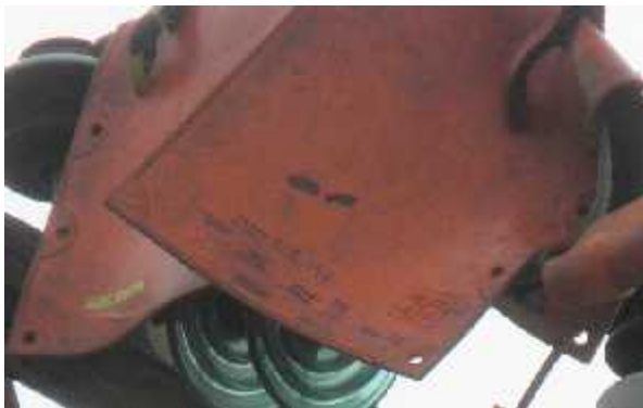
Insulating blanket in poor condition
