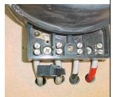
Where a risk of mistaken identification and connection may exist, eg, aging and discoloured VIR and/or TRS conductors, or neutral continuity relying on meter connections, the installations consumer mains neutral conductors must be identified by visual identification and testing and marked adjacent the terminations being worked on.
