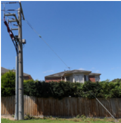
5 stay on a concrete pole
