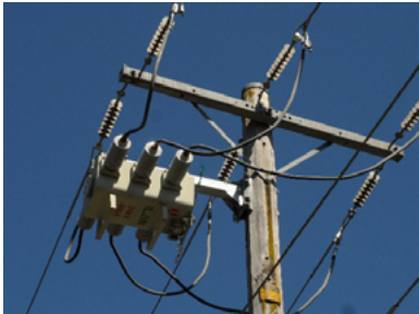
Two examples of gas switch mounting
