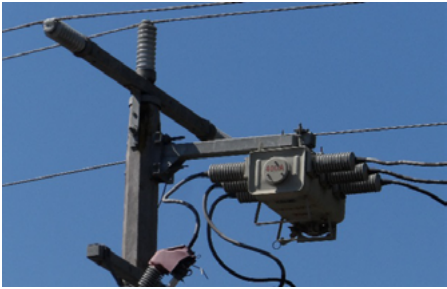
Two examples of gas switch mounting
